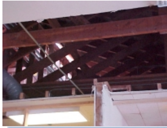
Main building attic area
