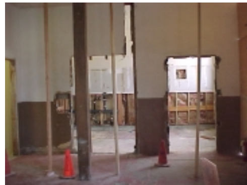
Main building classrooms
