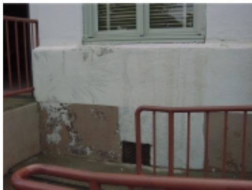
Exterior west side
