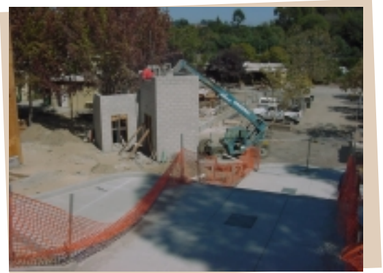
Construction of elevator structure
